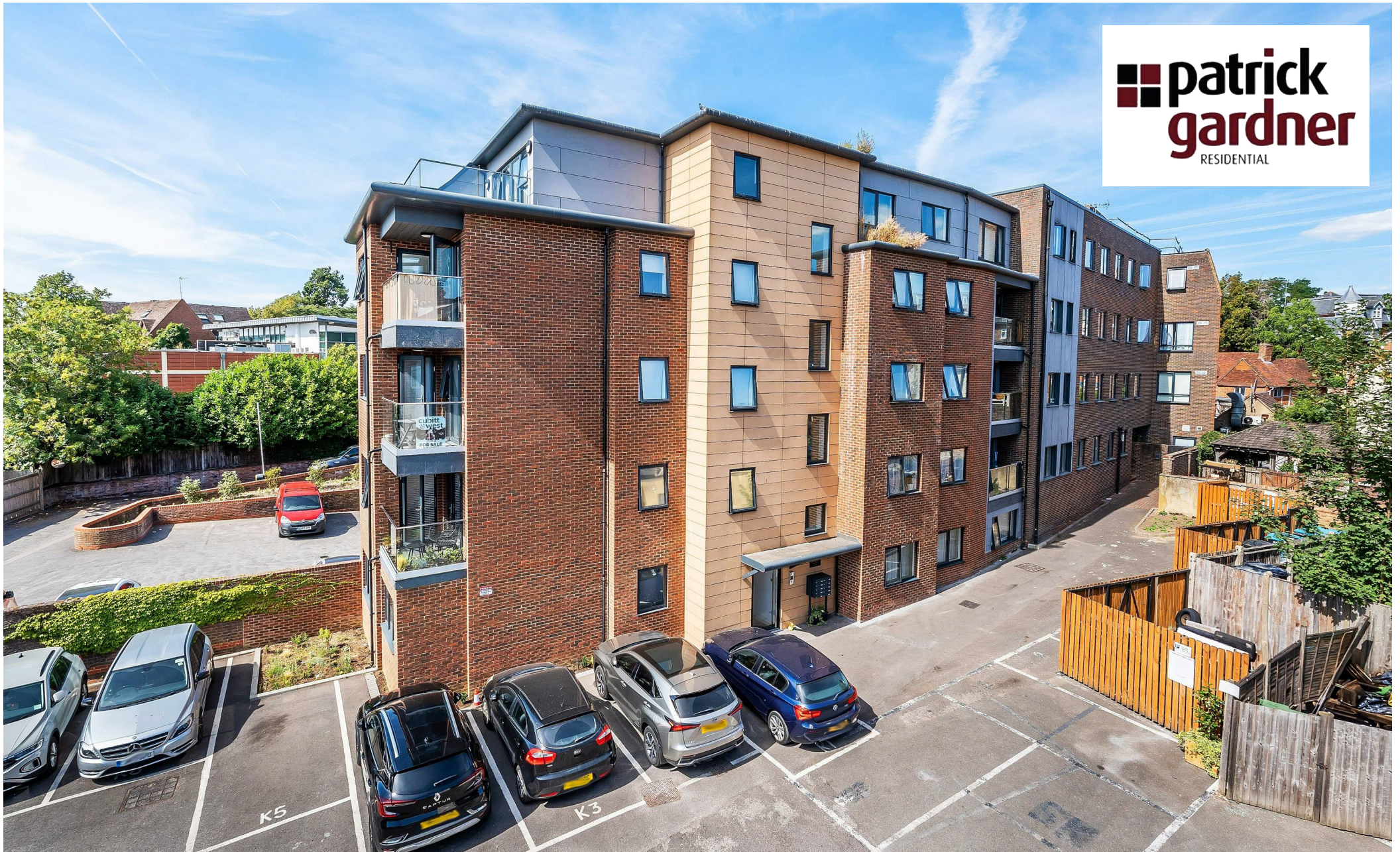
Flat 2, Kelsey Apartments 10A Bridge Street, Leatherhead, KT22 8FH
